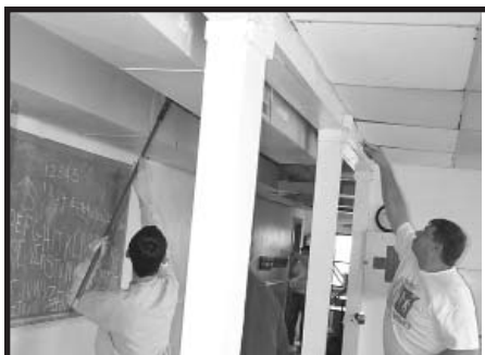
High ceilings and peeling paint made refurbishing Bldg. 203 a big job!
